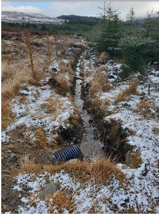
Photo 4. Ditch running inside northern fence line.
