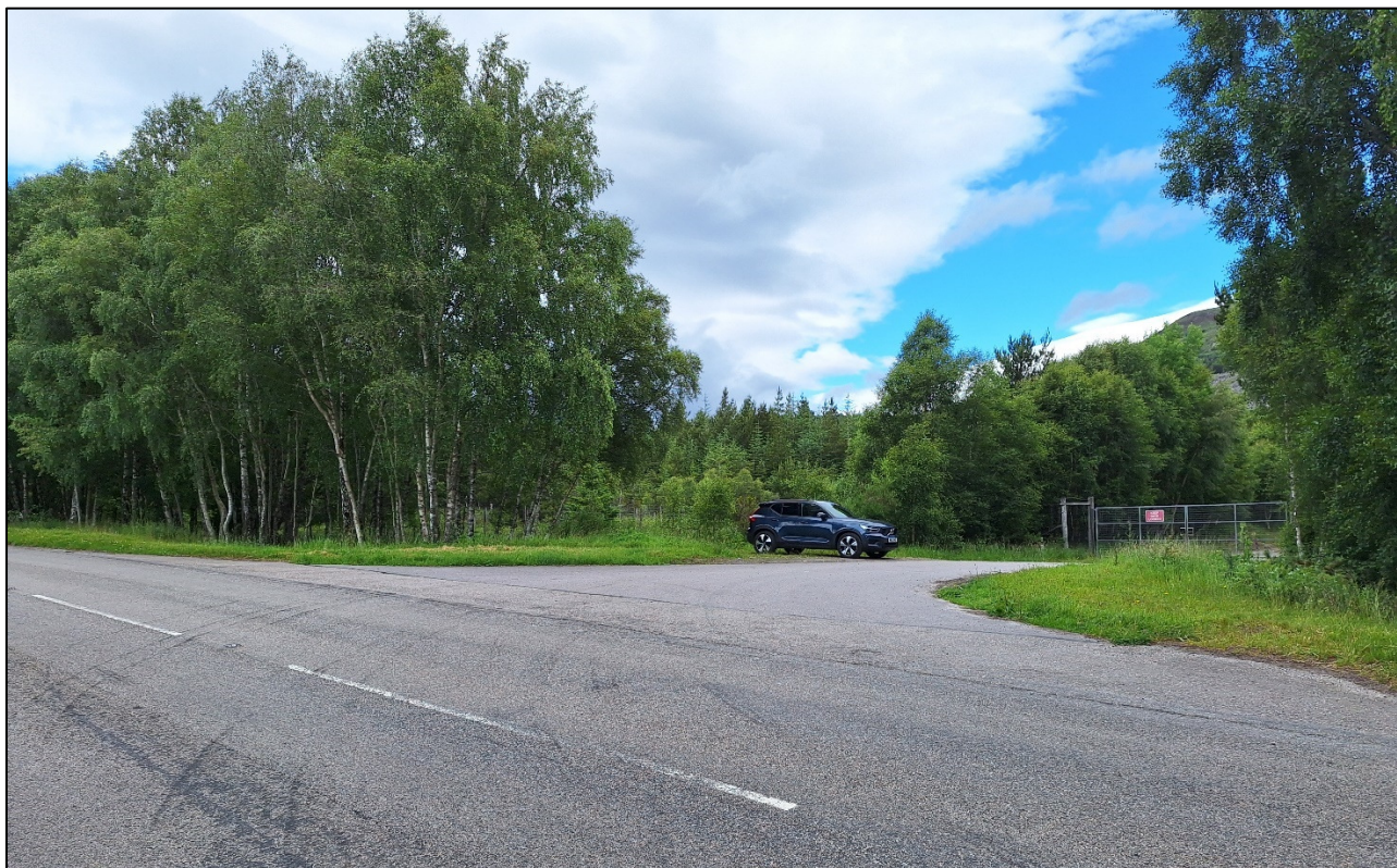
Figure 3 Existing Access Junction
